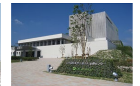
SAGA Heavy Ion Medical Accelerator in Tosu Kyushu International Heavy Ion Beam Therapy Center Saga, Japan (2013)
