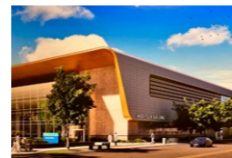
Mayo Clinic Rochester Campus *Additional construction Rochester, MN, USA (Under construction)
