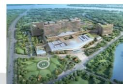
Heyou International Hospital Project Proton & Heavy Ion Center Foshan, China (Under Construction)
