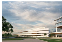
Mayo Clinic Jacksonville Campus Jacksonville, FL, USA (Under Construction)
