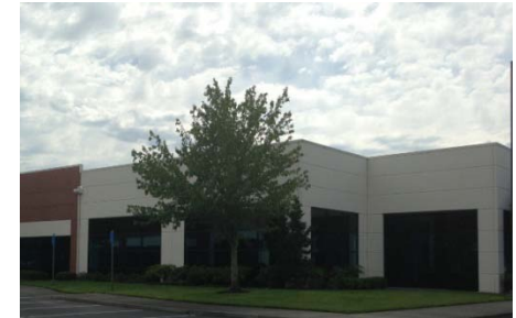
Process Engineering Center
