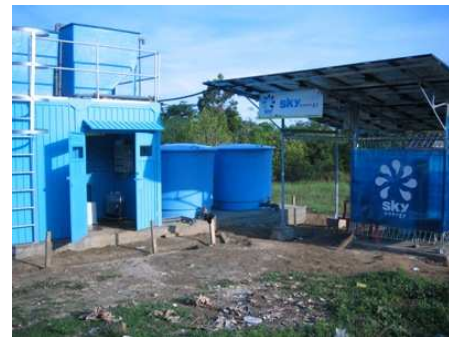
Village of Bekkae, in South Sulawesi, Indonesia Water purification system (left) paired with a solar power generation system (right)
