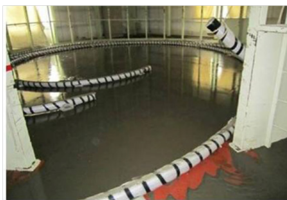
Fig.4 The high-voltage cable was damaged by the tsunami just before it was completed.
