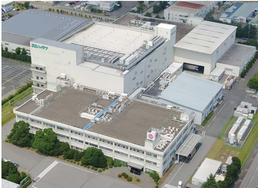
本社全景 Full view of headquarters
