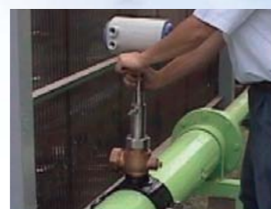
6. Insert the flowmeter into the pipe.
