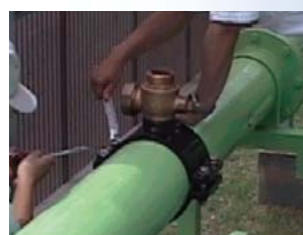
1. Secure the corporation stop with saddle on the pipe.
