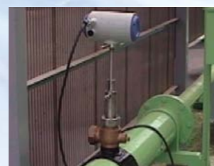
7. Check the wiring and operation.
