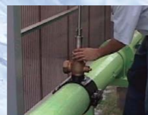
4. Install the flowmeter.
