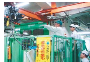
■ Safety diagnosis by the Central Association for Prevention of Labor Accidents
