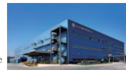
Exterior view of the new factory
